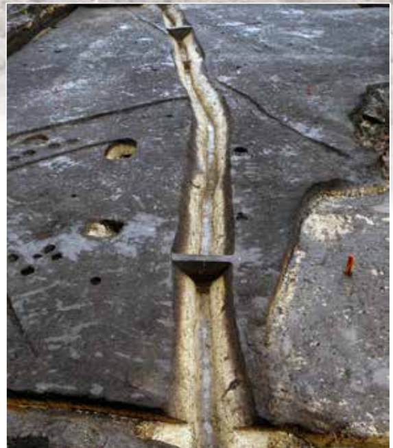
V字溝 Ditch with a V-shaped profile
